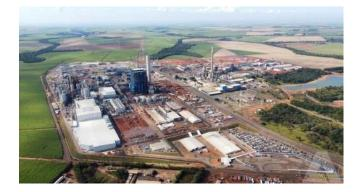
by Andritz on an EPCC (Engineering, Procurement, Construction, and Civil Construction) basis. Four chipping lines, two stacker-reclaimers, eight chip screening units, biomass handling with two Andritz BioCrushers, and biomass storage are among the features.
