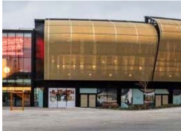
Picture 5: The way in which their properties combine predestines them for façade or ceiling projects, here as a façade cladding of the type PC-Alu 6010 of Elwick Place in London.
